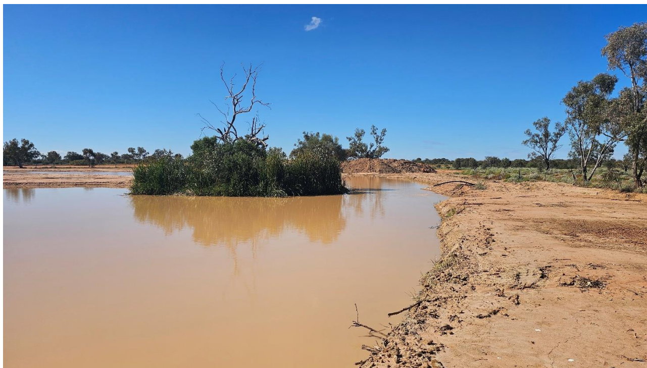
Golf Course – Desilted effluent ponds 1 and 2
