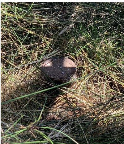
Leaking bore head
