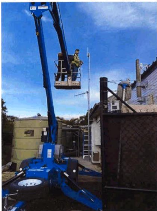
Installing a gateway at a Vacuum Pump Station
