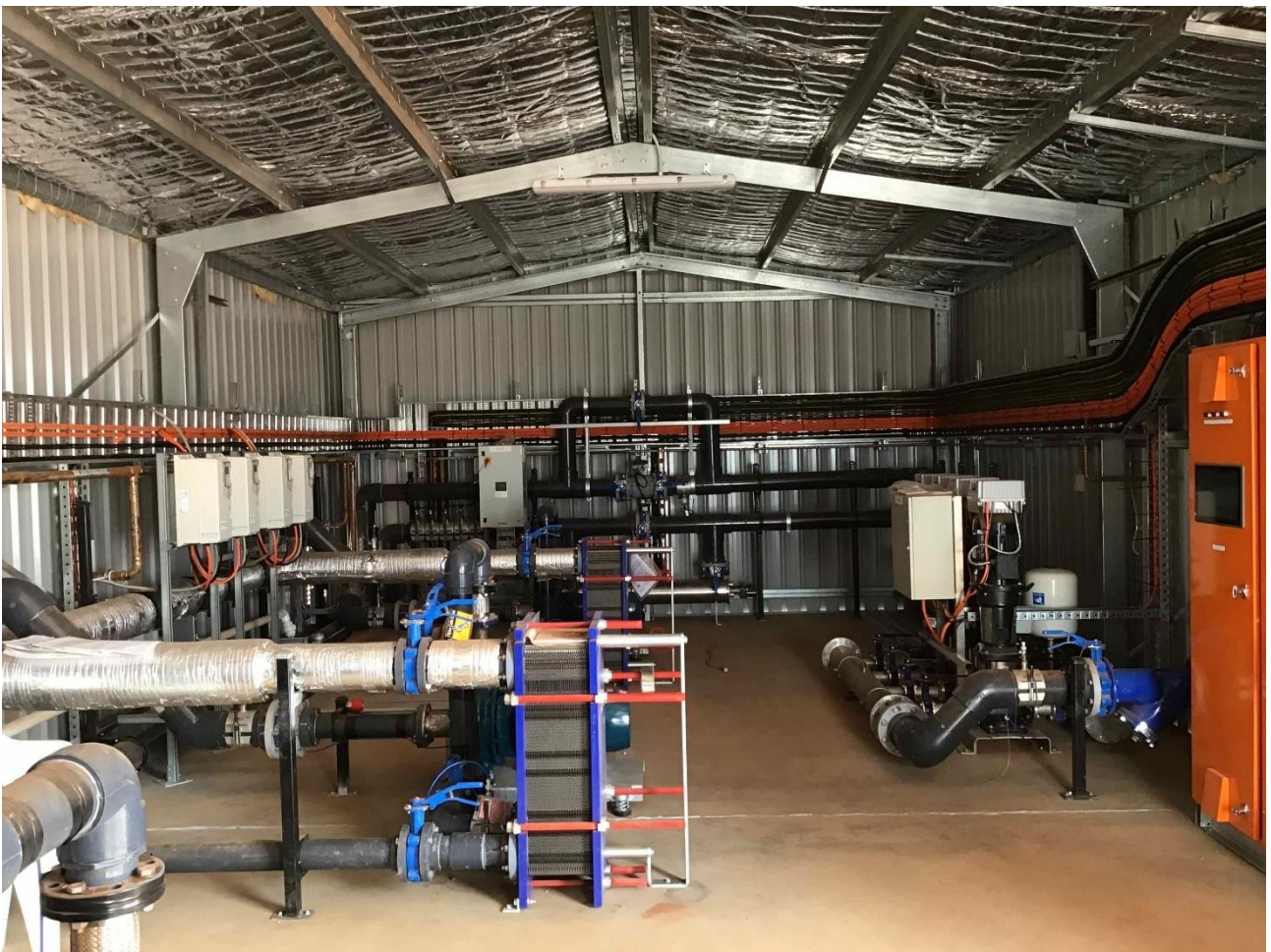
Thargomindah's Heat Exchange Unit – the secondary cooling system.
